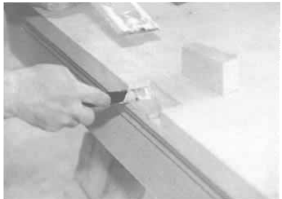
4 Make certain that the contact surfaces of repair stone will fit the slot. Then, butter the squared hole with epoxy mixed for the purpose.
