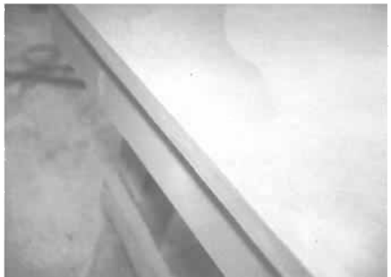
8 The completed repair will be nearly invisible.
