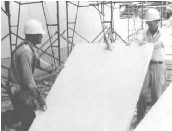
Lifting stone panels from horizontal to vertical with clamp or other top-only attachment can cause breakage and injury.
